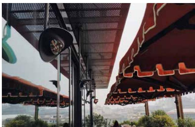
Another example of customization was the request from a Hotel to have longer poles for hotdoor ceiling mounted. The aim was to heat the tables without standing in the way of the sun umbrellas. In this case our technical staff developed one-meter-long poles and a custom fixing capable to stand against the strong winds of the rooftop.
